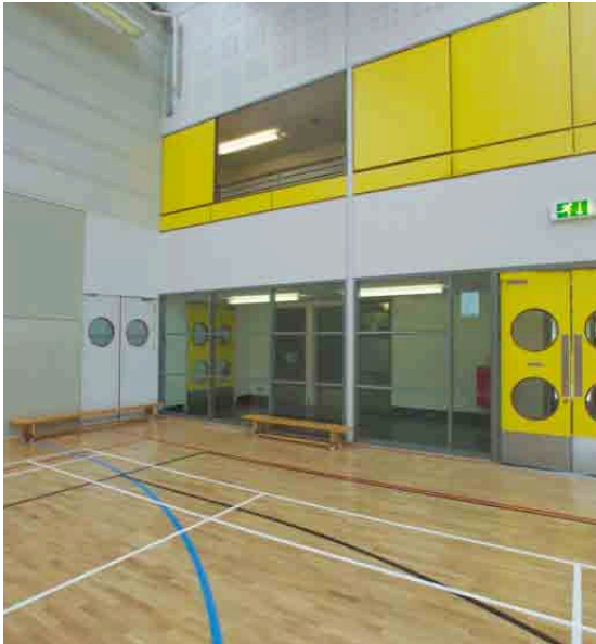
Screen panels fitted to first floor viewing to give privacy
